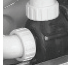
Vent air by slightly opening pump unions.
