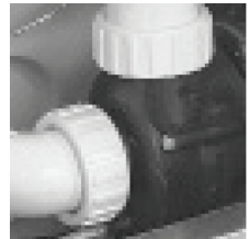
Vent air by slightly opening pump unions.
