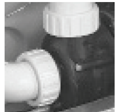
Vent air by slightly opening pump unions.
