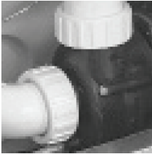
Vent air by slightly opening pump unions.
