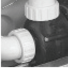
Vent air by slightly opening pump unions.
