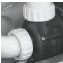
Vent air by slightly opening pump unions.
